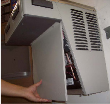
Remove Front Panel
