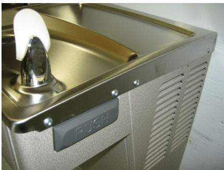
Remove Basin Fasteners
